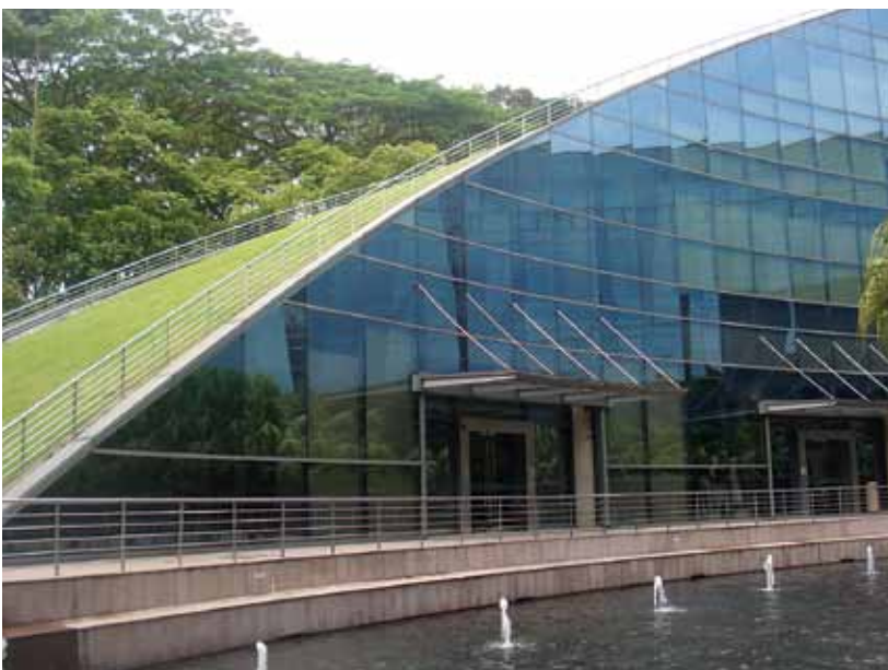
A steep green roof at a university.
